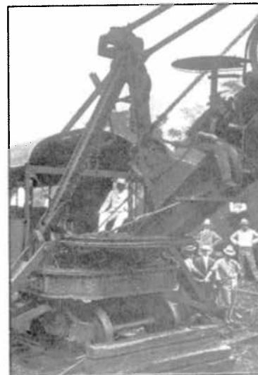
President Roosevelt works a steam shovel at the canal.
